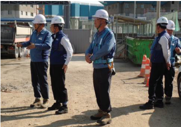
CEO’s health and safety check at a housing site in Wirye
